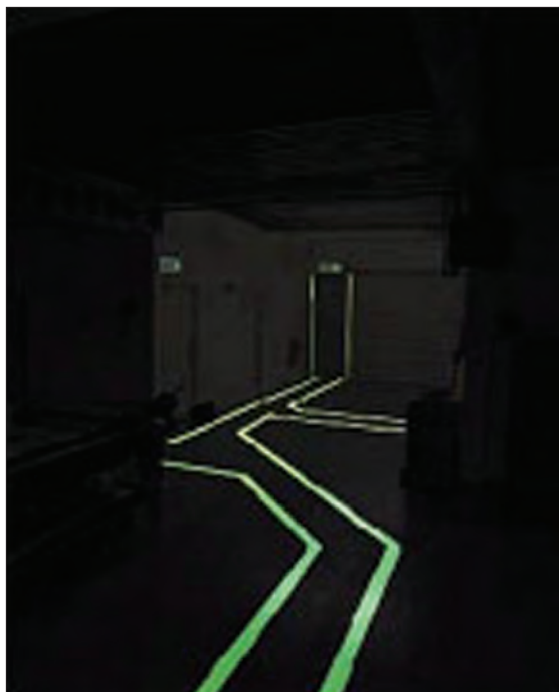
Figure 56: A way-guidance system
